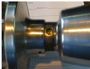
Slide the knob off the spindle (notice the poke holes in both the knob and the rose)
