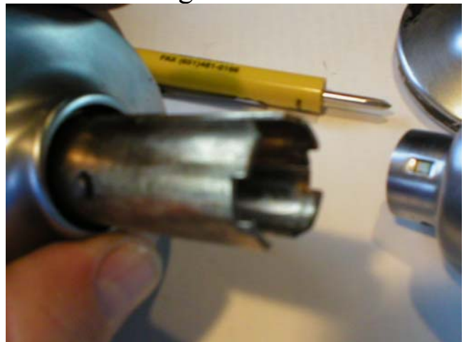
Notches on spindle that keeps the faceplate from being removed while on the lockset.
